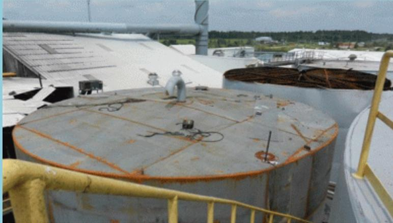
**An explosion of what was thought to be nonhazardous materials blew the top off of this tank, killing one worker and severely injuring another**
