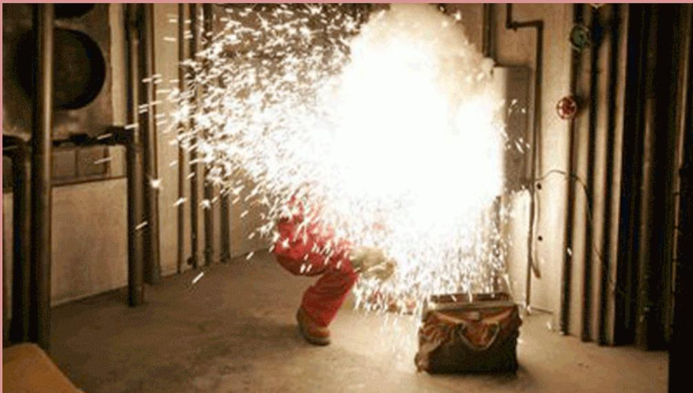
Arc flashes in electric equipment are hazardous to workers and can result in fatalities, costly damage to equipment and delays in production until repairs are made. Arc-flash labels on electrical equipment are required by federal law; OSHA regulations requiring these labels have existed since approximately 2000.
